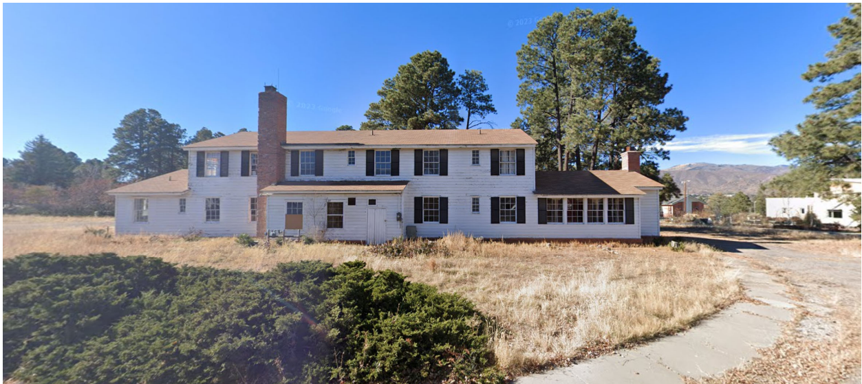
Image 1: Google Earth Street Image, Nov. 2022 – Women’s Dorm Building east elevation facing 17 th Street
