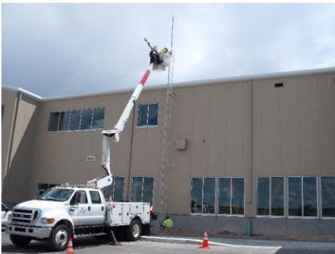
Pajarito Cliffs Site Radio Tower Install
