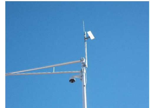
Typical Intersection Install
