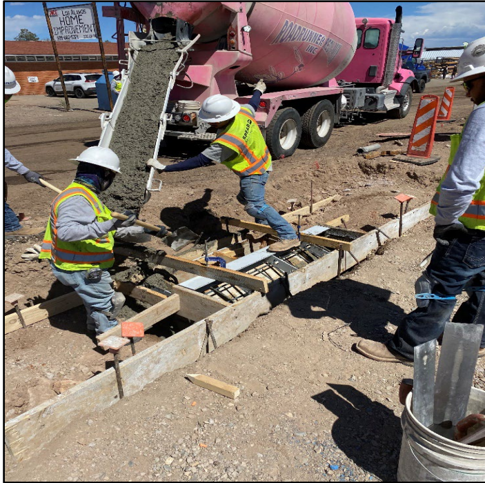
Concrete operations continue, as crews install new stormwater inlets and a new curb and gutter from Cross Fit Gym west toward the Fire Station.
