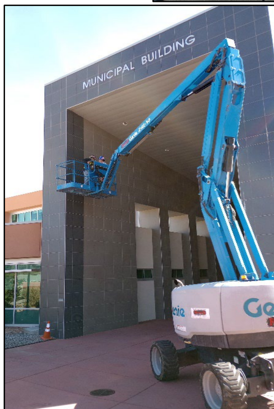
Facilities crew perform a thorough tile condition inspection at the main entrances to the Municipal Building.
