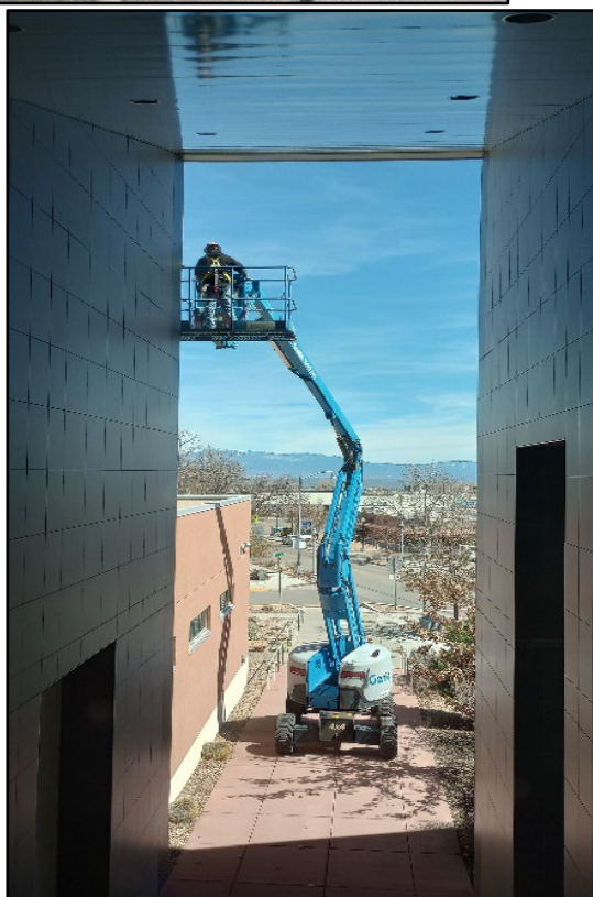
Facilities crew perform a thorough tile condition inspection at the main entrances to the Municipal Building.
