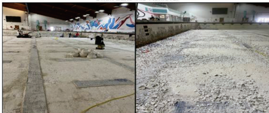
Finished Plaster Removal
