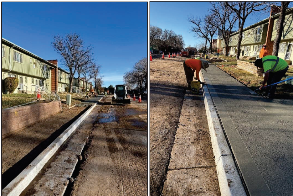
ADA ramps, curb and gutter and sidewalks along 9th Street.
