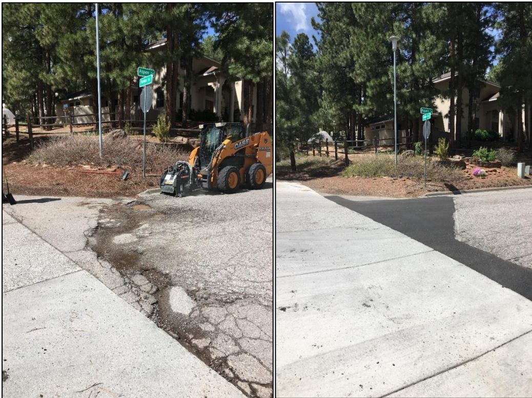
Crews repaired a bad intersection at the entrance to Ponderosa Estates.
