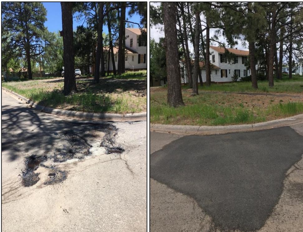
Crews repaired potholes on North Sage per a work request.
