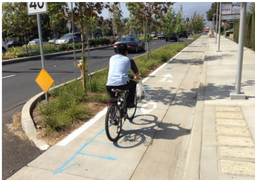
Figure 3.3: Bike lane separated by buffer with green and trees on Rosemead Boulevard, Temple City, California.
