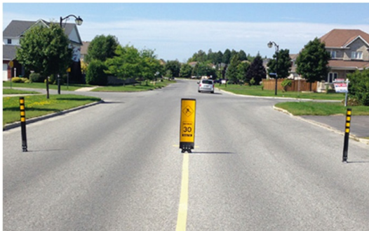
Figure 3.14: Side and center bollards on Kittiwake Drive, Ottawa, ON. These bollards reduced the 85% speed from 35 mph to 25mph without narrowing the road [8].
