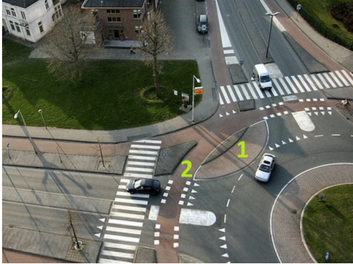
Figure 3.11: This roundabout has the disadvantage for a straight entry for cyclists onto the road. This leads to higher cyclist speeds and increases accident risk.
