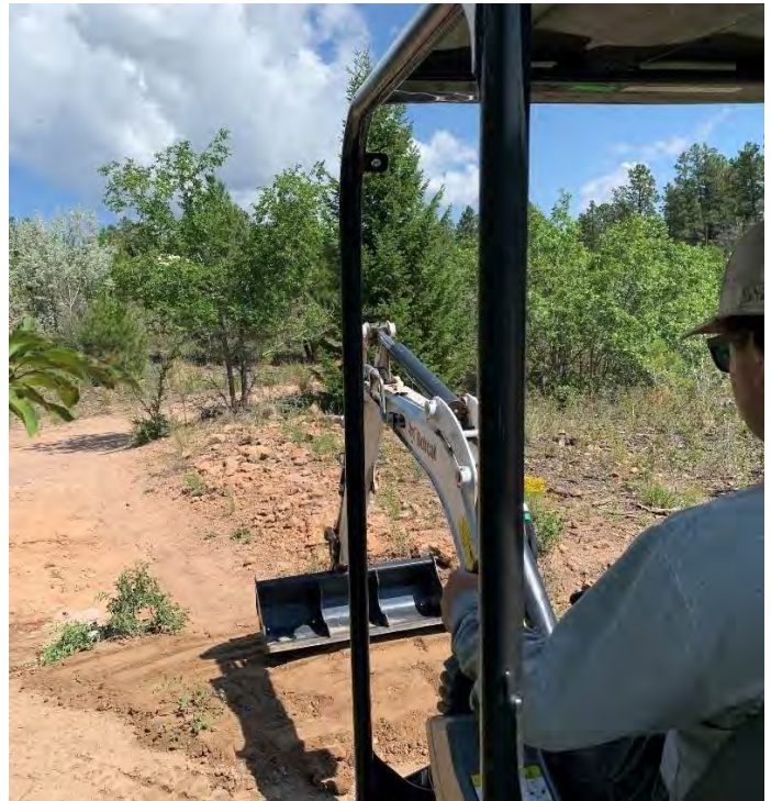
Building water bars at Quemazon trailhead.
