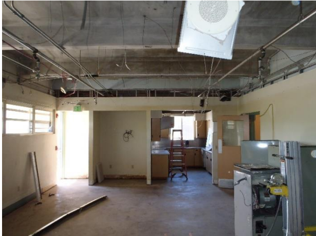
FS4 Day Room – Demolition
