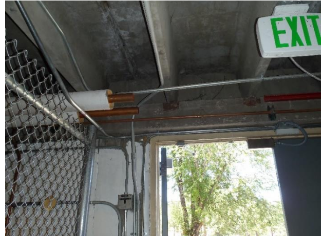
Basement Heating Piping Cut off for New Loop
