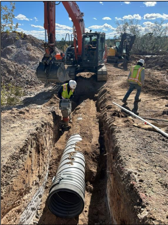
DP Road Improvements Project
