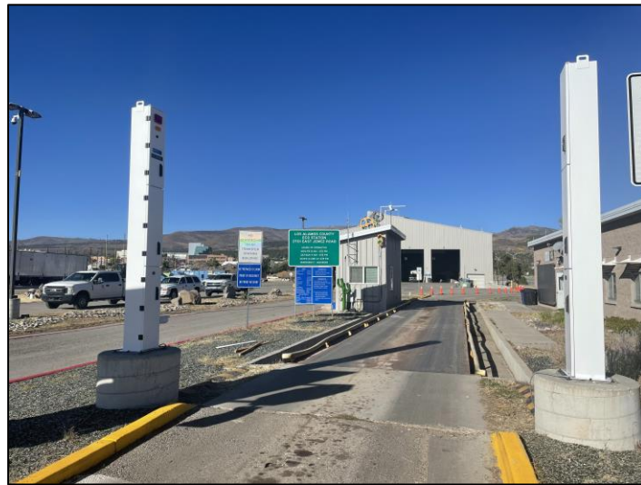
Upgraded Portal Monitors
