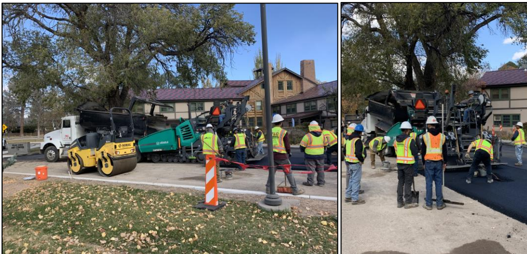
Paving – Bathtub Row Project.
