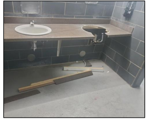
Repair's at Ashley Pond Restrooms
