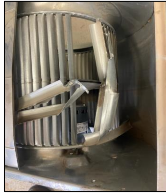
Bayo Plant Heater Repairs
