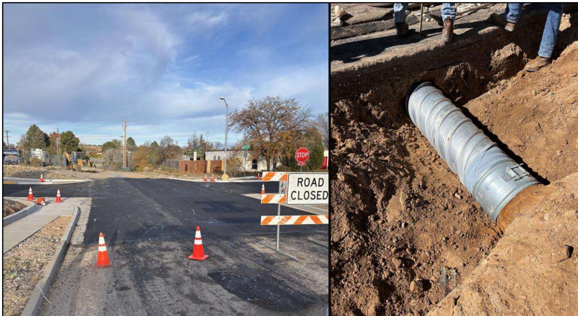
Streets crews excavated, prepared and laid asphalt and repaired a culvert that eroded at the intersection of Aragon and Cheryl Avenues.
