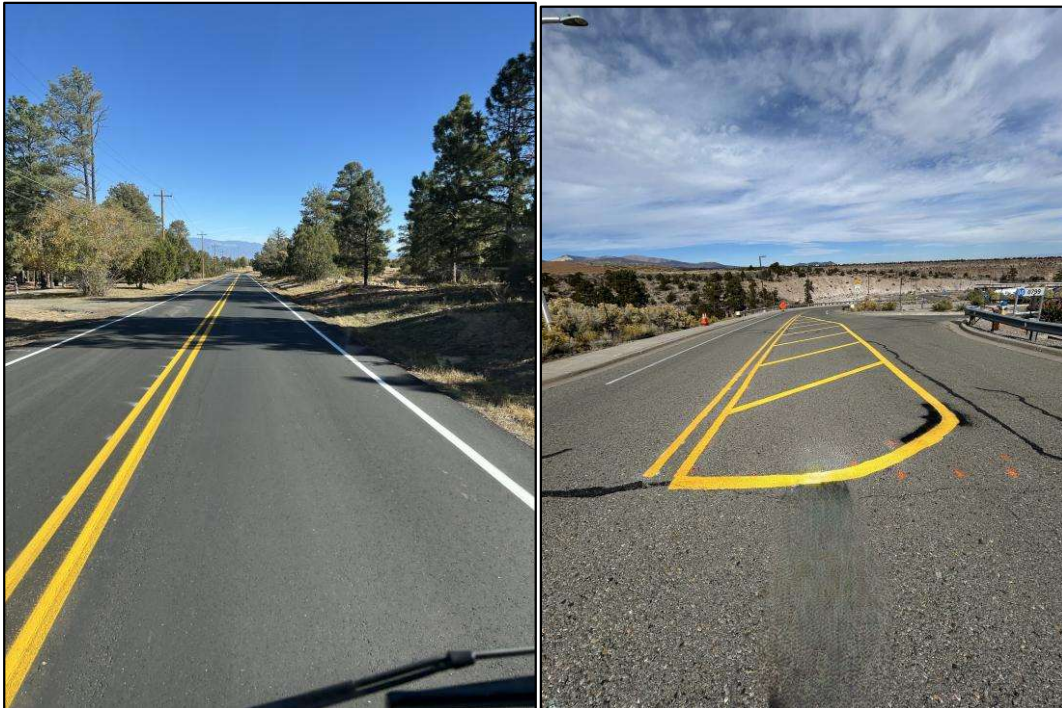
Signs and Markings crew striped paved sections on San Ildefonso Road and Camino Entrada.
