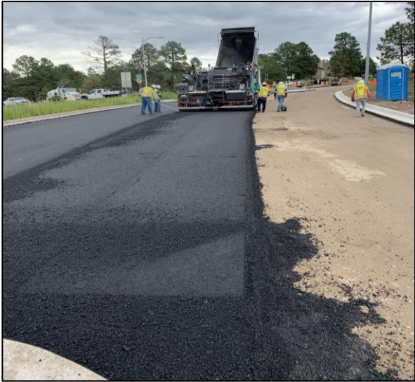
Canyon Rd. Road & Utility Improvements
