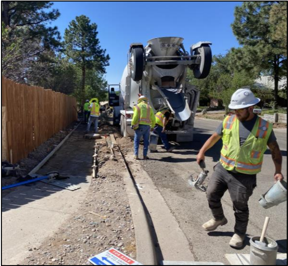
Cumbres del Norte Roadway & Utility Improvements
