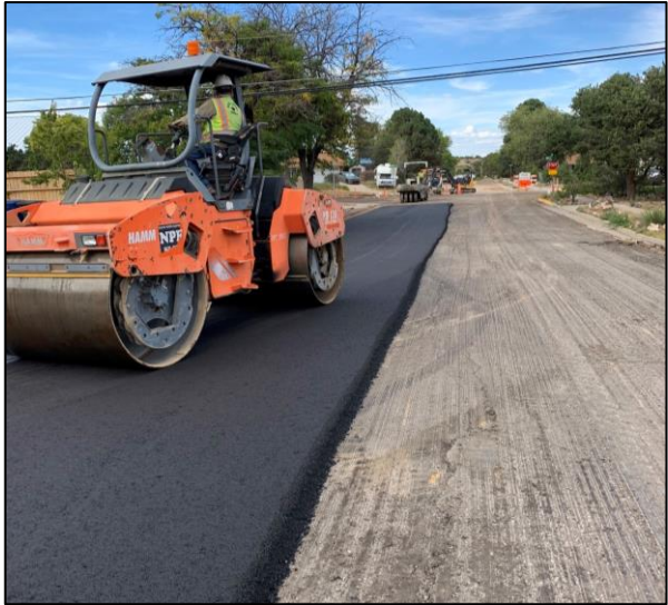
Sherwood Blvd. Road & Utility Improvements
