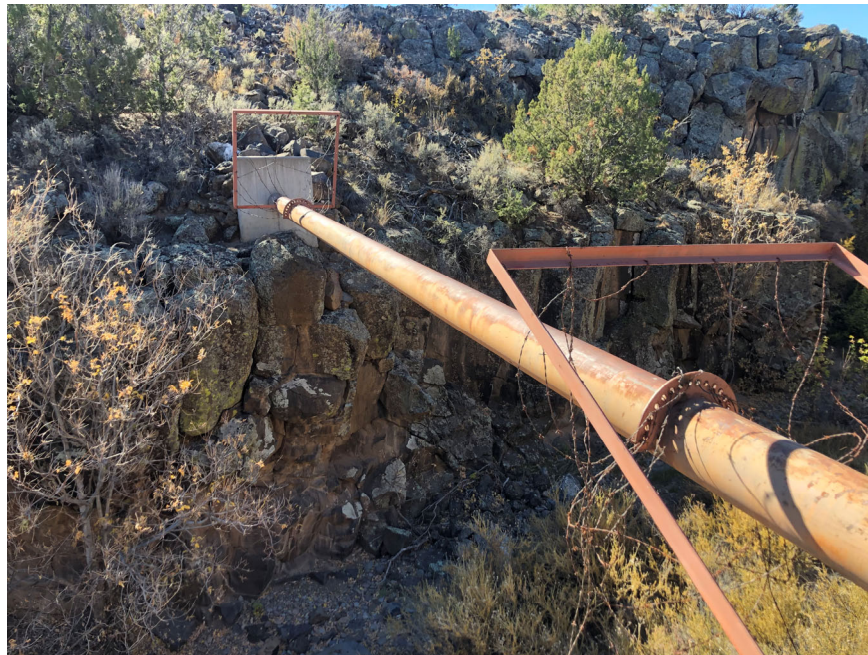
Figure 25: Pajarito Force Main Crossing Looking South
