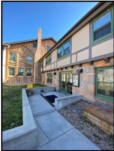
View of drains at entry and concrete retaining walls
