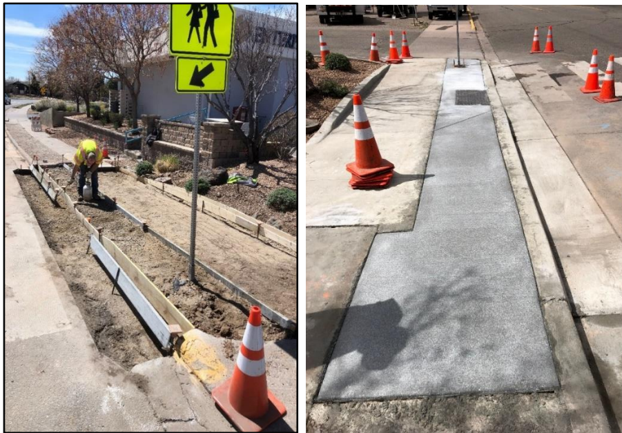
Crews installed a new ADA ramp at the cross walk on Rover Blvd. and Meadow Ln. in White Rock.
