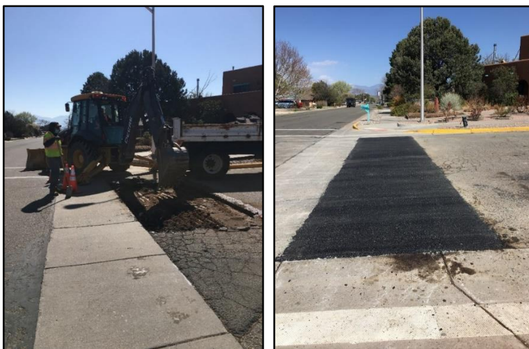
Crews performed Pavement Preservation in-house and patched a large section of failing asphalt on Aragon Ave. in White Rock.
