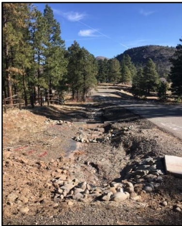
Crews repaired and placed erosion protection on a drainage channel at Ponderosa Estates.
