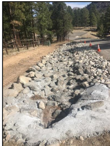
Crews repaired and placed erosion protection on a drainage channel at Ponderosa Estates.
