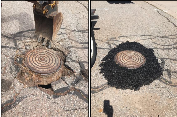
Crews temporarily fixed manhole at Mesa Vista Dr. in White Rock
