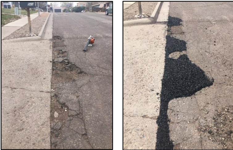
Crews repaired a section of broken asphalt on Alamo Drive.
