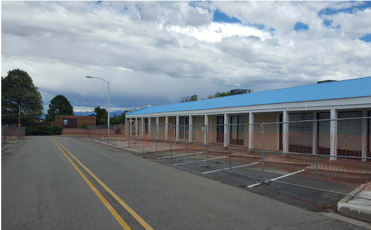
Figure 5. Office building along Longview Drive that was recently demolished due to multiple issues with the building.
