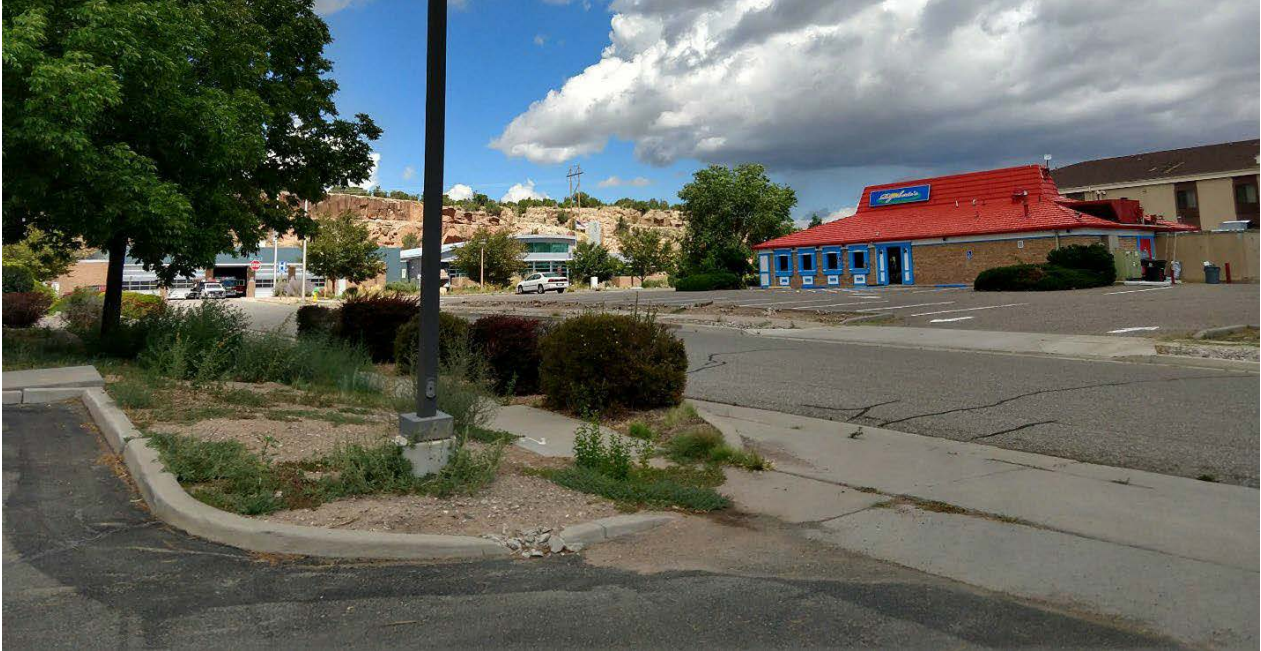
Figure 8. Degraded site improvements and overgrown landscaped areas along Bonnie View Drive.
