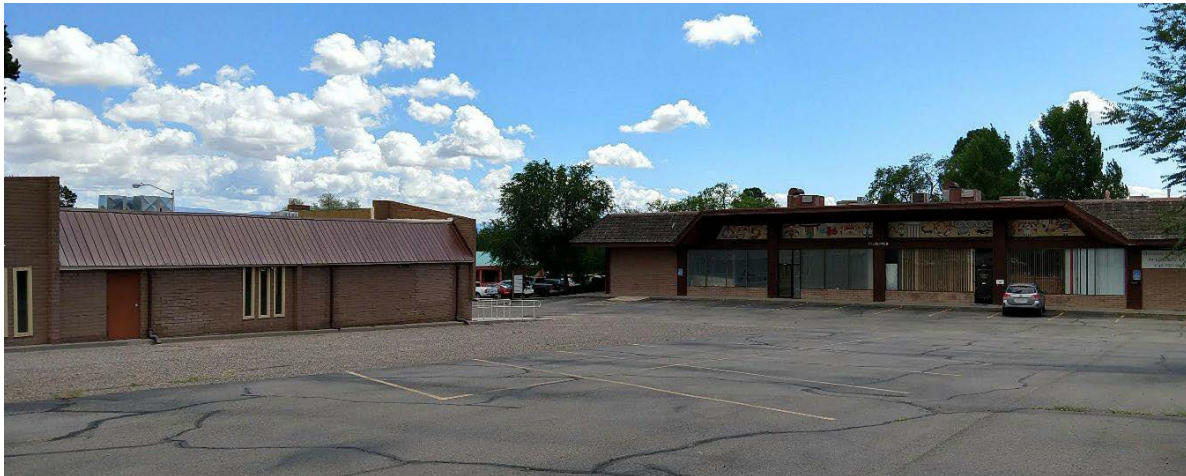
Figure 2. The White Rock Business Plaza site, which currently has several vacant storefronts and buildings that are outdated and need improvements to attract new tenants.
