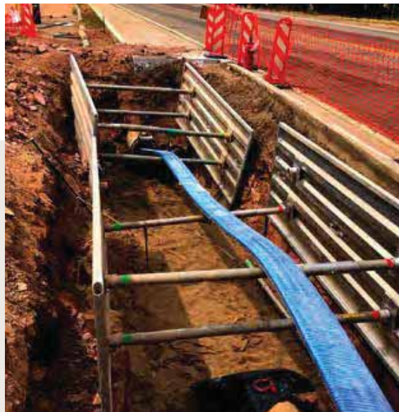
16-INCH WATER LINE INSERTION PROJECT ON PAJARITO ROAD.
