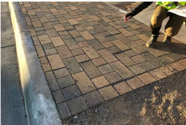
Permeable pavers allow water to infiltrate the soil instead of contributing to runoff, Albuquerque, NM
