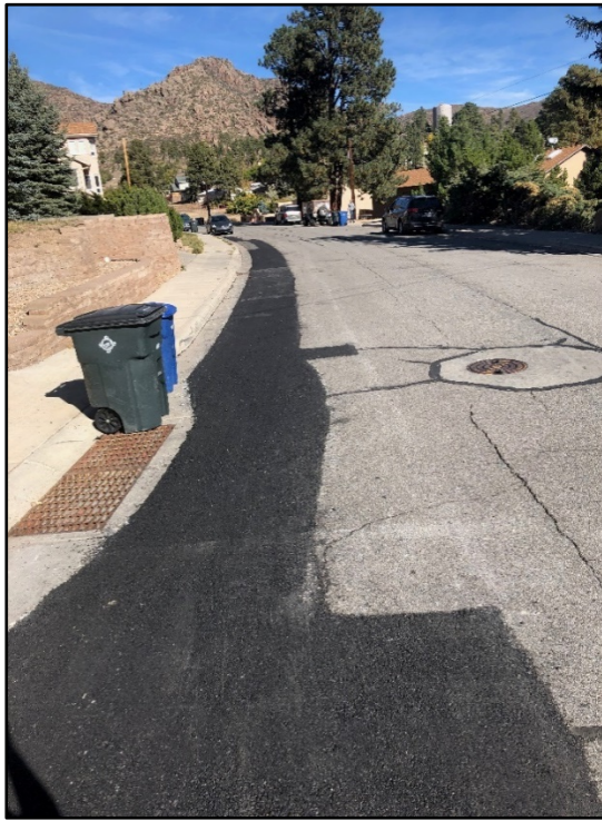
Crews milled and replaced a section of asphalt on 45 th Street near Yucca Drive.
