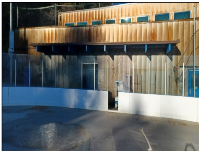
Ice Rink gutter install. We had new gutter installed on the new building so water does not drip on spectators.
