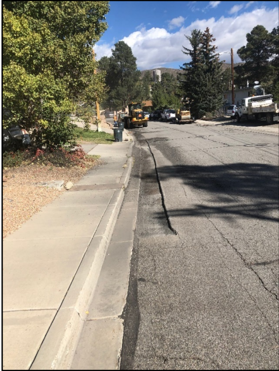
Crews milled and replaced a section of asphalt on 45 th Street near Yucca Drive.
