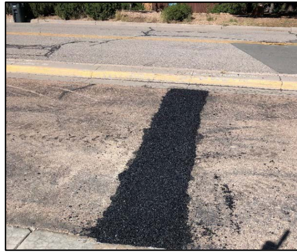
Crews patched asphalt on the bus lane at Barranca School.
