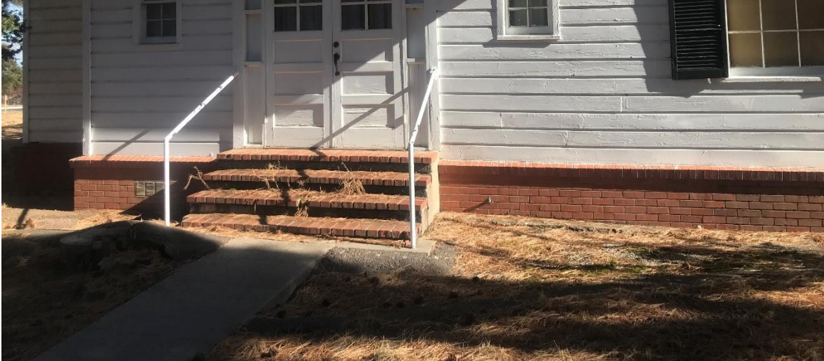
Figure 3-13: Foundation Brick Veneer Source: Mueller Heller Architecture
