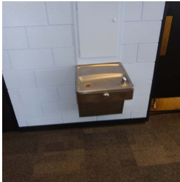
Noncompliant fountain and aging door hardware
