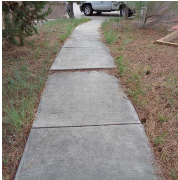
Noncompliant access walk with trip hazard
