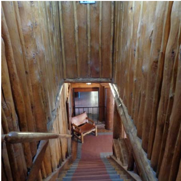
Access stair with noncompliant handrail
