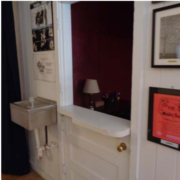
Noncompliant fountain and Dutch door transaction counter
