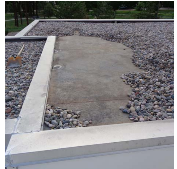
Old ballasted roofing with aggregate removed
