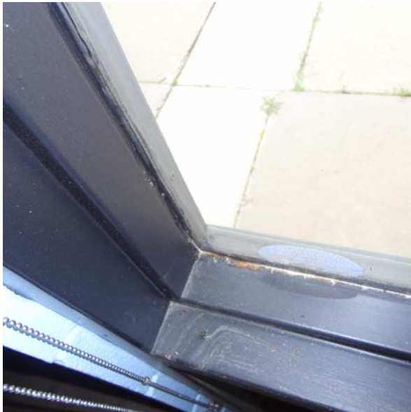
Leaking noninsulated window and rusty frame
