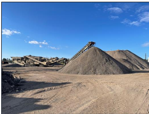
Crushed Concrete at Eco Station
