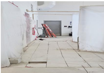
Lagoon Closure for Concrete Repour
