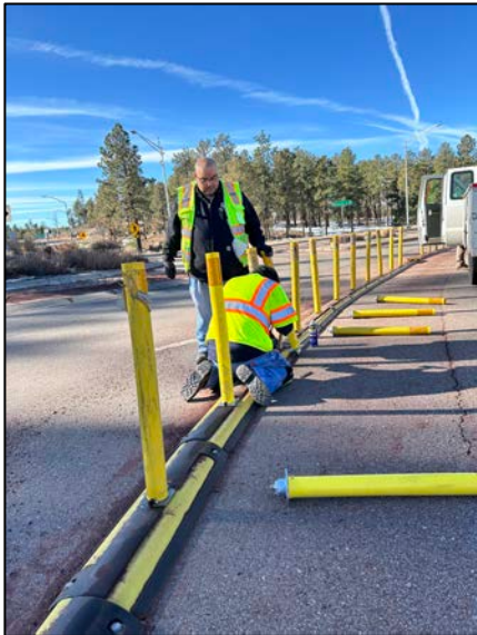
Replacing tube delineators at the Diamond Dr. roundabout.
