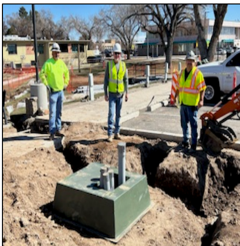
Progress at the Ashley Pond electrical upgrade project. Photos show the newly installed electrical pedestals for use by food trucks. First photo shows the location of one of the electrical transformers on site.
