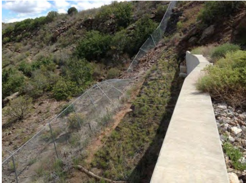
Figure 4.32. Debris/Fence Damage at Airport
