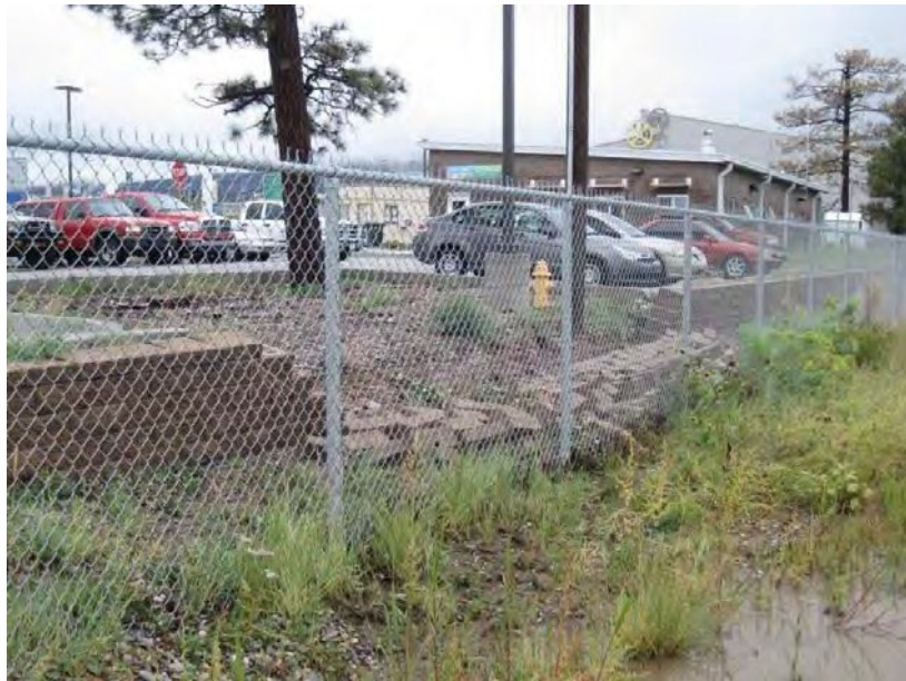
Figure 4.31. Damage to Retaining Wall at ECO Station
