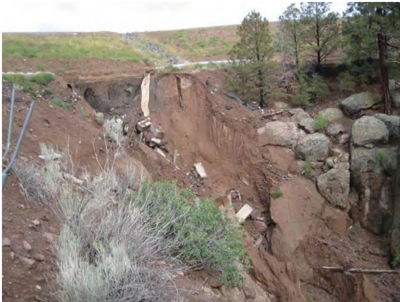
Figure 4.29. Landfill Sedimentation Pond Erosion
