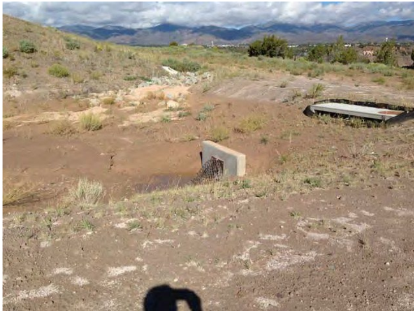
Figure 4.29. Landfill Sedimentation Pond Erosion
