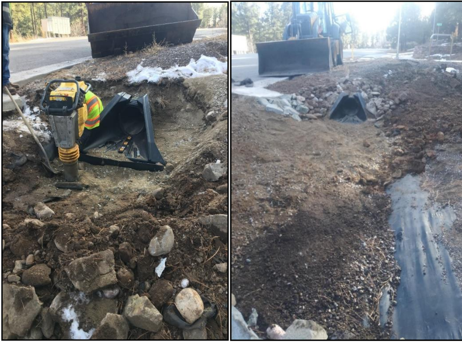
Crews installed drainage outfall protection at Ponderosa Estates drain.
