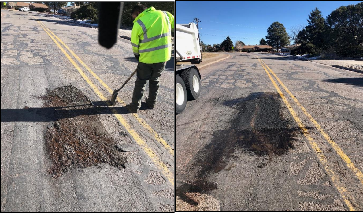
Crews worked on asphalt patching on Barranca Road.
