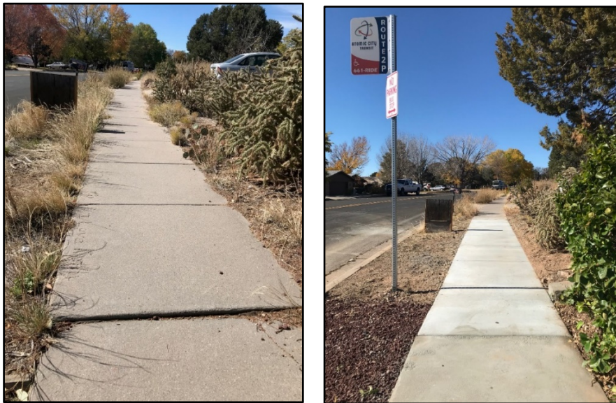
Before and after of sidewalk repair and removal of a tripping hazard in White Rock.
