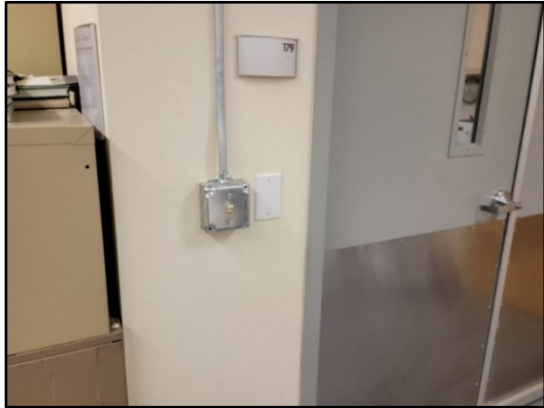
Added light switches to archives vault.
