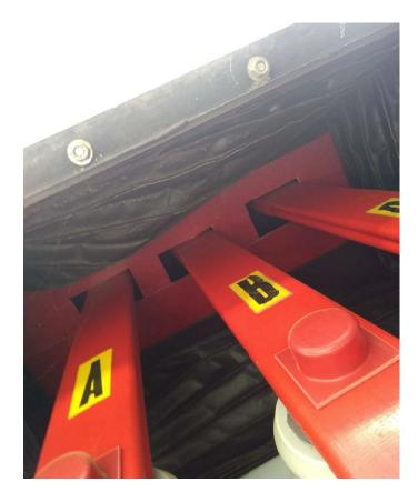
Boot Section and existing bus duct to be reused for new LV transformer connection.
