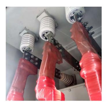
LV Transition Compartment Showing bus connections and linkages along with support insulators and LV bushings.
