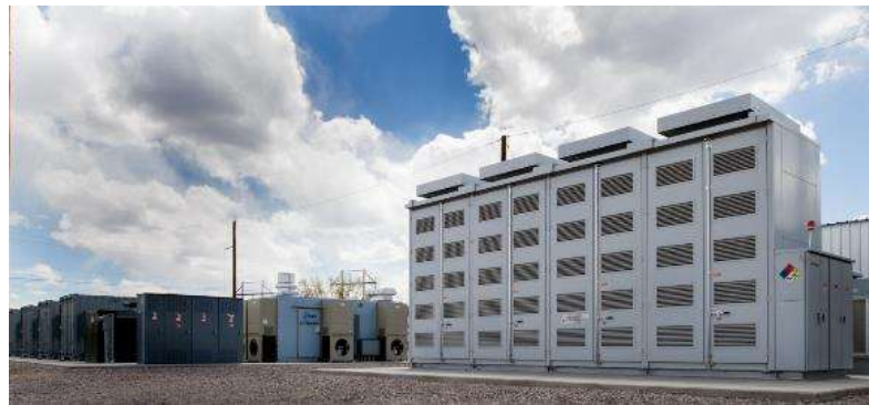
1-MW x 6 MWh NaS battery
