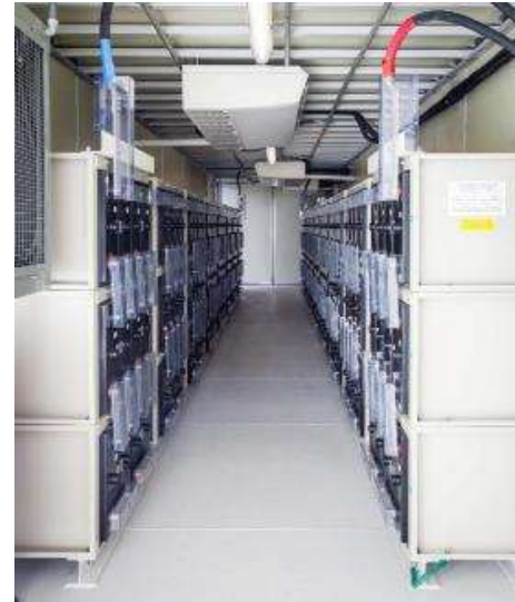
800 kW x 2.3 MWh lead-acid battery
