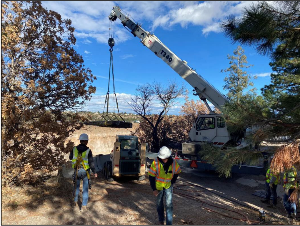
Catwalk Removal at the Airport
