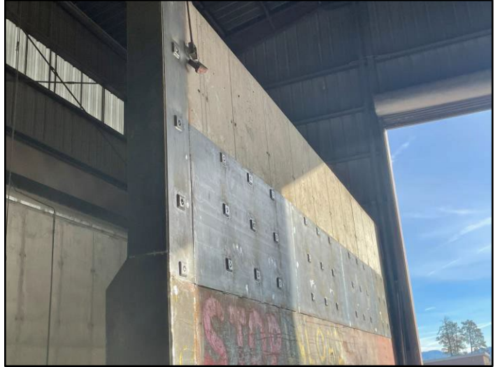
Transfer Station Wall Repair
