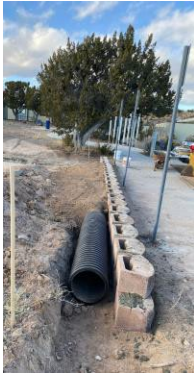
Wall Being Built at White Rock Branch Library to Control Erosion
