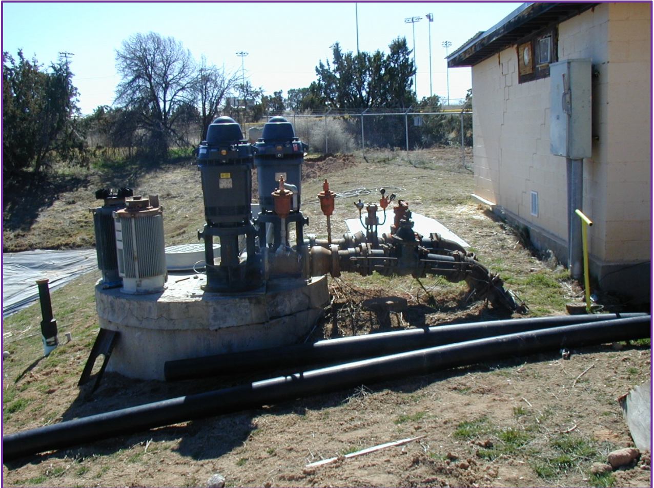
Photo of existing booster pumps installed in 1982.
