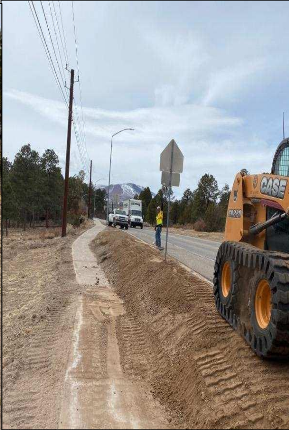
Crews placed material and built back up the shoulders on North Mesa.
