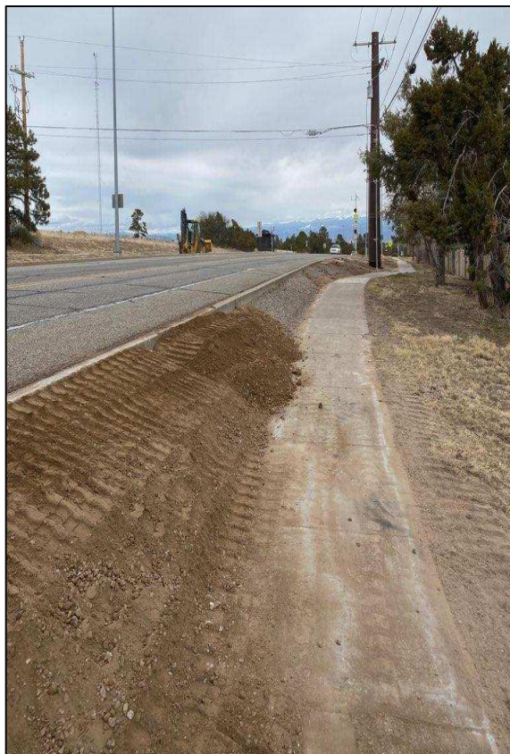
Crews placed material and built back up the shoulders on North Mesa.
