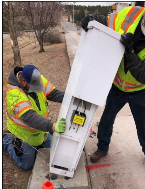
Crews replaced the street lighting meter that was damaged by a crash on Diamond in front of the Fire Station.
