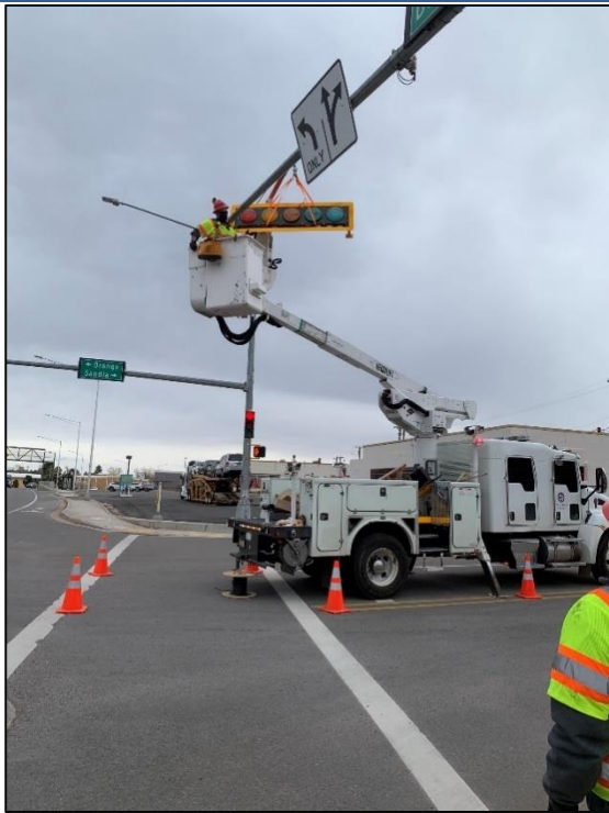
Crews installed a new signal head at the Diamond/Sandia intersection. The new signal head has left turn phases that will improve traffic flow at this intersection.
