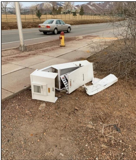
Crews replaced the street lighting meter that was damaged by a crash on Diamond in front of the Fire Station.
