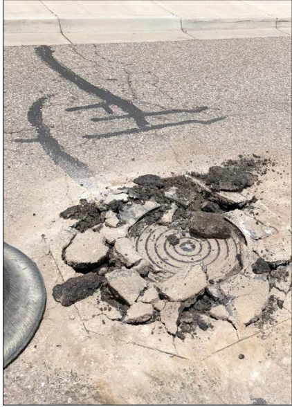
Crews removed and replaced concrete around manholes on Aztec in White Rock.
