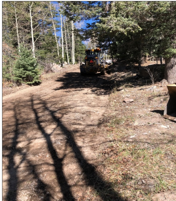
Crews worked to repair the shoulders along Ski Hill Road.
