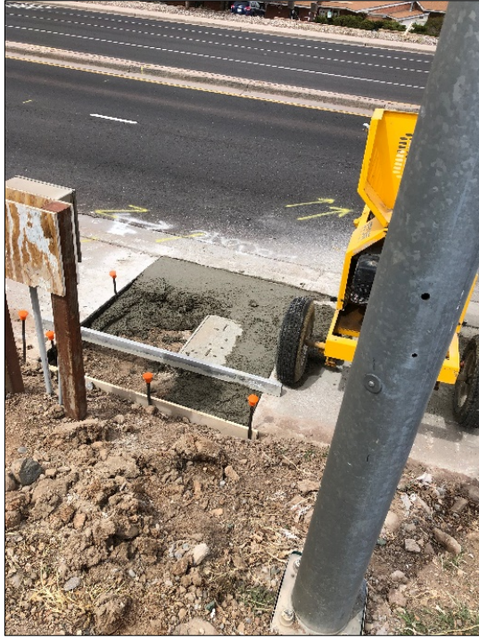
Crews replaced a section of sidewalk on Trinity Drive after the relocation of a utility box.
