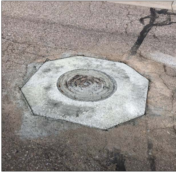
Crews removed and replaced concrete around manholes on Aztec in White Rock.
