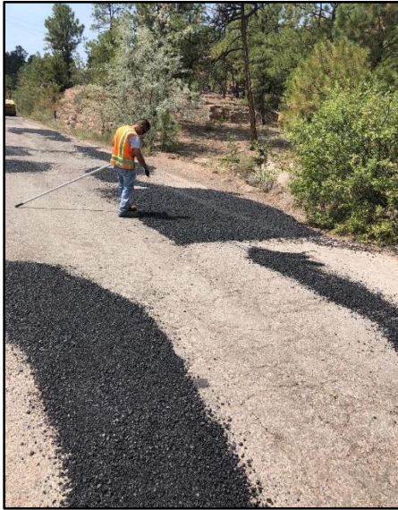
Crews patched sections of asphalt on Rendija Canyon Road.
