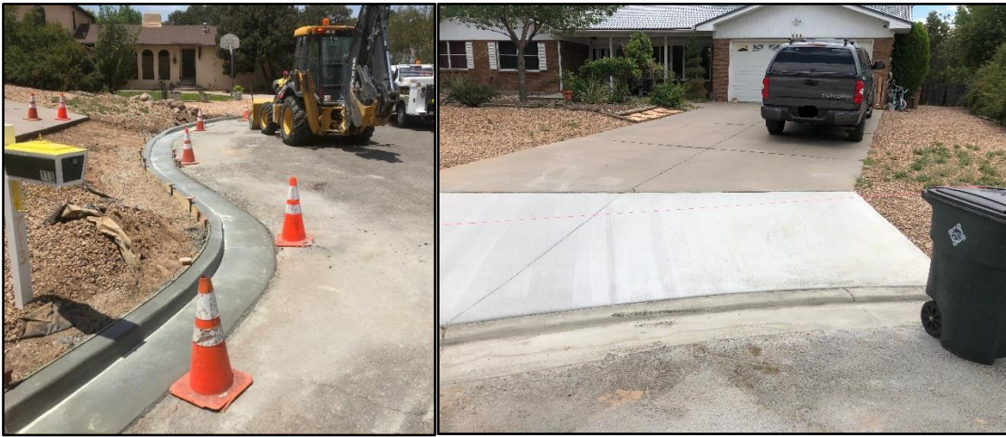
Crews replaced a drive pad and gutter on Kris Court.
