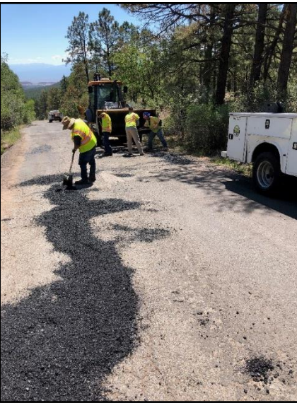
Crews patched sections of asphalt on Rendija Canyon Road.
