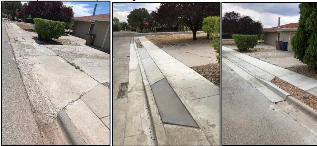
Crews replaced a drive pad, gutter, and sidewalk on Kimberly.
