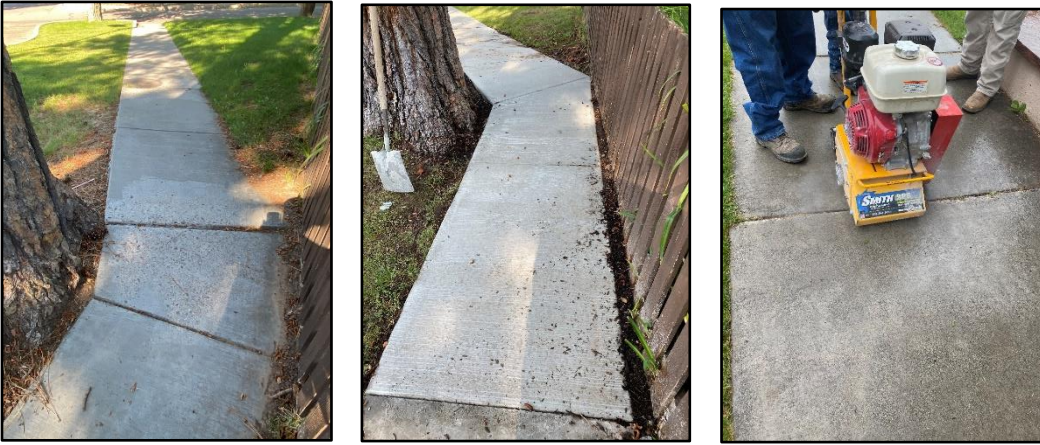
Crews repaired sections of sidewalk and removed trip hazards near Fuller Lodge.
