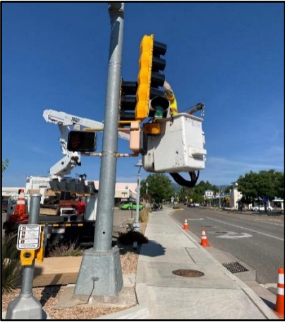
Traffic electricians changing out traffic signal heads at Central/15 th .
