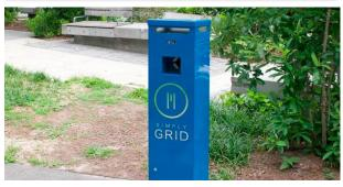
Simply Grid supply easy access to grid electricity for food trucks.
