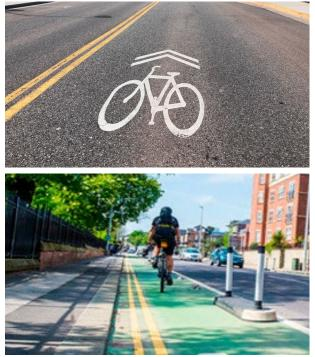
TOP: A pavement marking known as a "sharrow" BOTTOM: A bike lane with pavement marking
