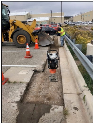
Crews repaired a section of the parking lot at Pajarito Cliffs site where a sink hole was identified.
