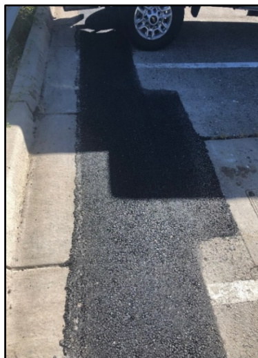
Crews repaired a section of the parking lot at Pajarito Cliffs site where a sink hole was identified.
