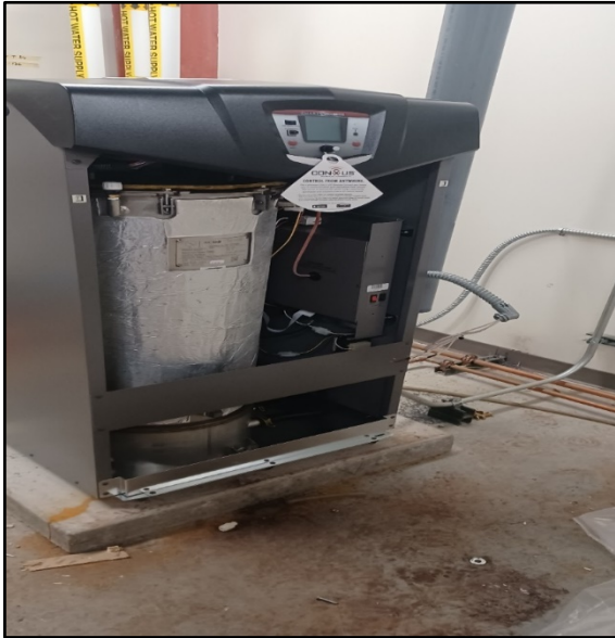
PCS-1 – Replaces boiler for Heating loop for VAV Boxes
