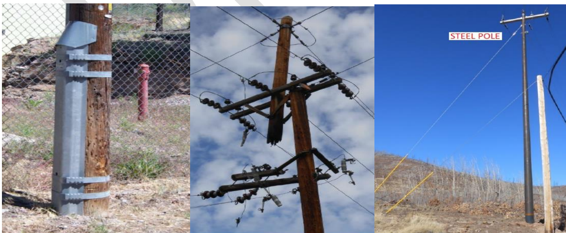
Figure 14. Typical braced pole & backbone broken pole; & new Steel Pole
