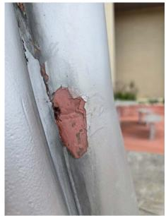
Detail: Area of failed paint pulled back to a stable point prio to painting
