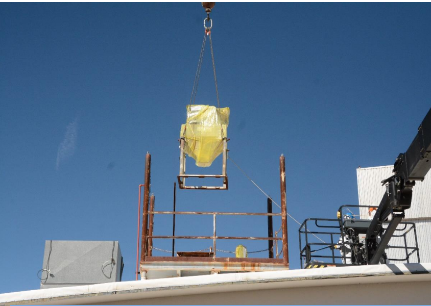
Large Equipment Removal
