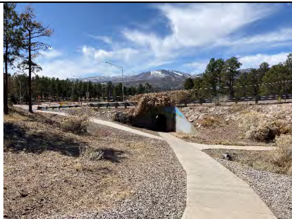
Connection to San Ildefonso ped underpass
