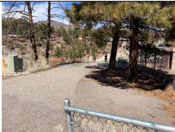
Paved drive leads to trail access
