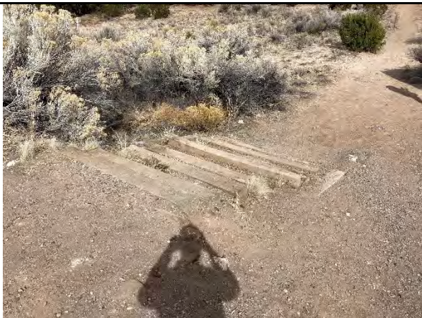
Existing stairs from street to trailhead
