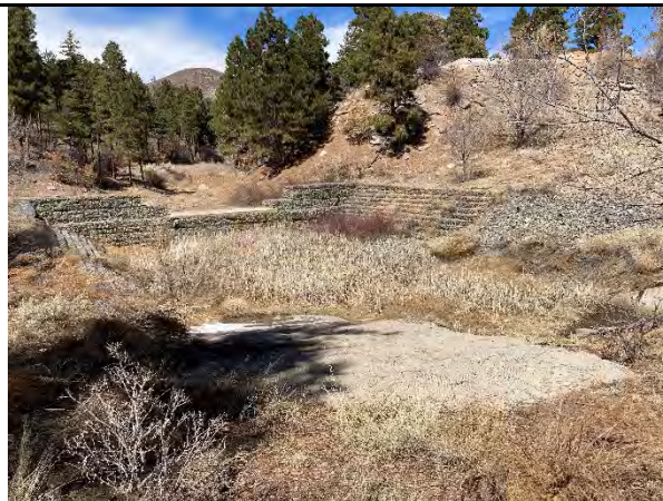
Drainage feature just beyond access point
