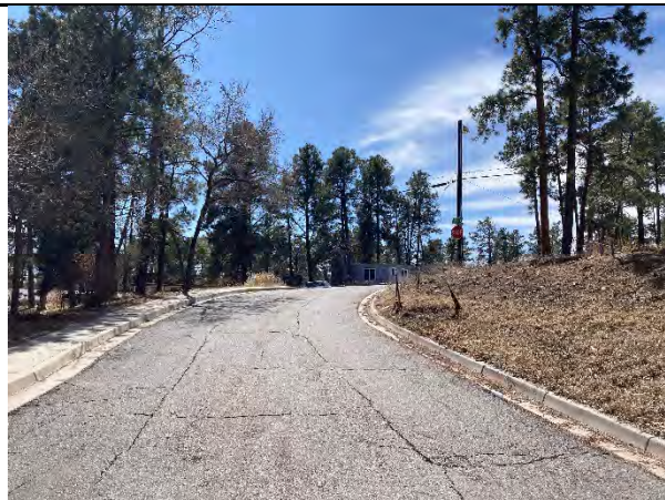
Access road looking up from tennis court
