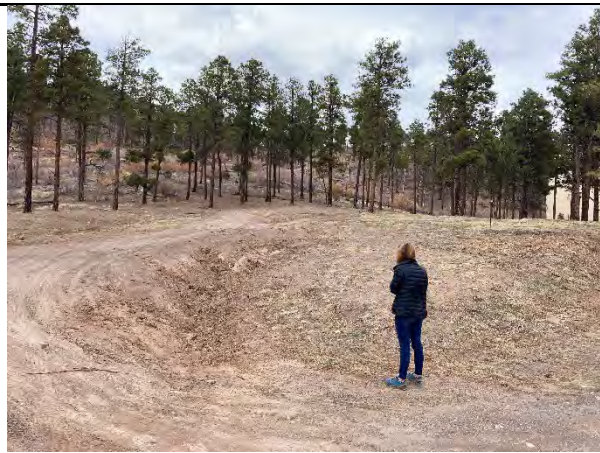
Access road/trail; lack of trail signage
