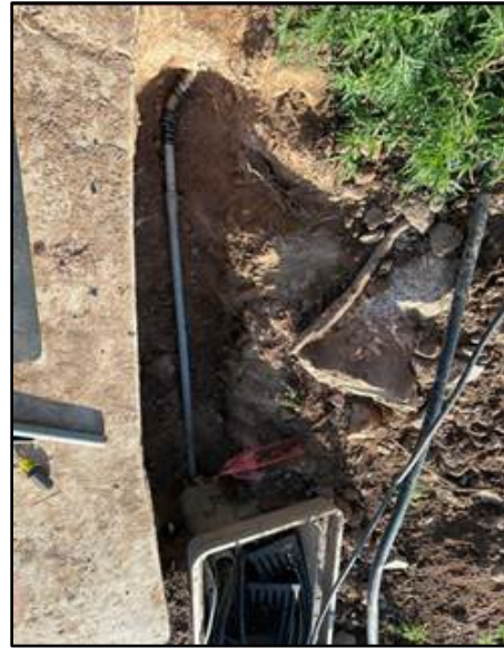
Traffic electrician trenched and installed conduit and relocated an exposed streetlight feed on Sioux St.
