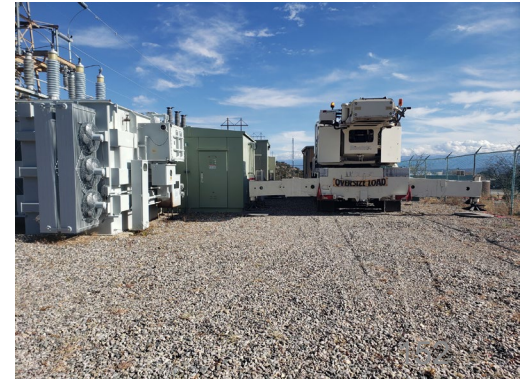
White Rock Transformer Replacement
