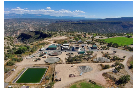
White Rock Water Resource Reclamation Facility
