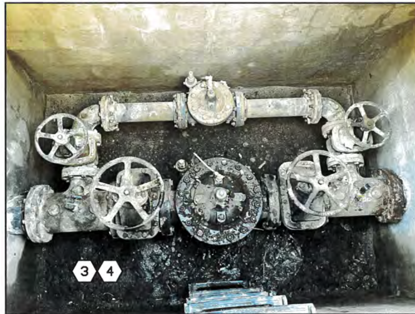
C 17 BROADVIEW PRV VAULT SCALE: NTS
