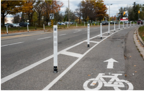
Figure 3.2: Bike lane with buffer created by paint and bollards [7].
