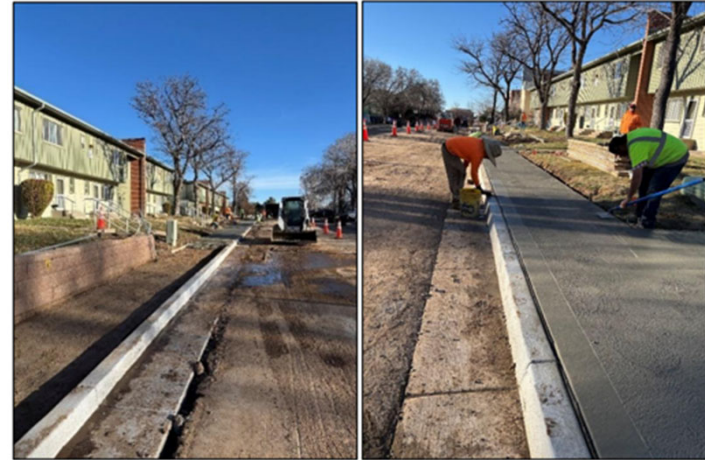
ADA ramps, curb and gutter and sidewalks along 9th Street.
