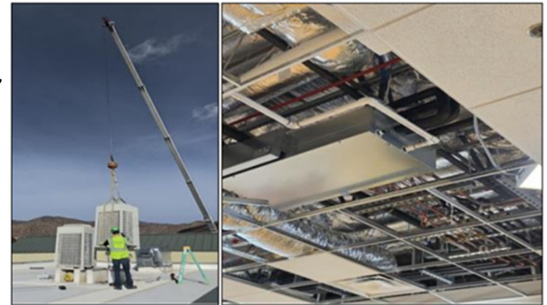
Removal of existing HVAC system and installed new units inside and in the roof of the Clubhouse Community Room.
