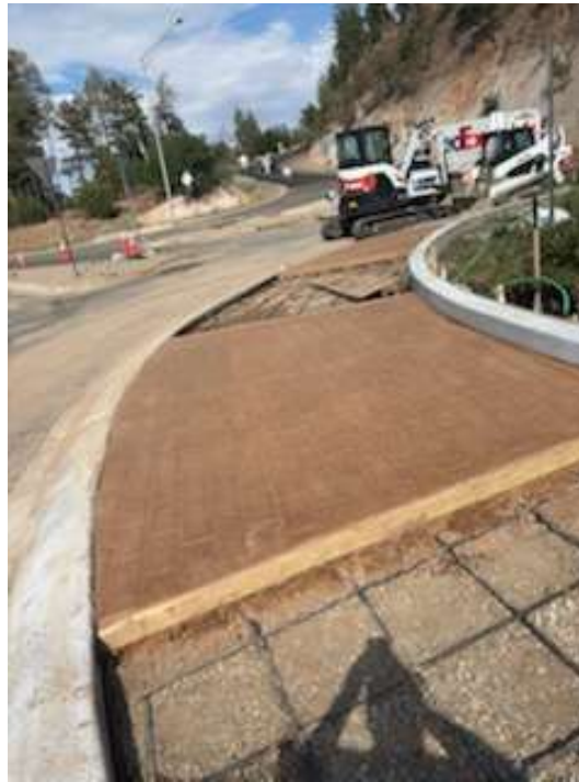
San Ildefonso Roundabout Truck Apron
