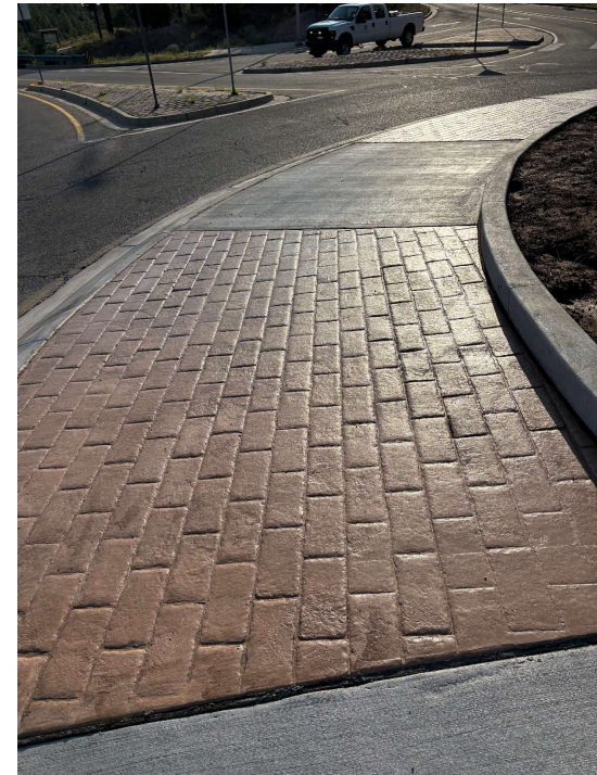
San Ildefonso Roundabout Truck Apron
