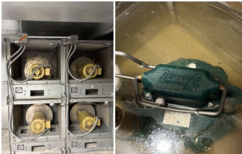
White Rock Library Pump Replacement and Mesa Library Motor Repair and Replacement
