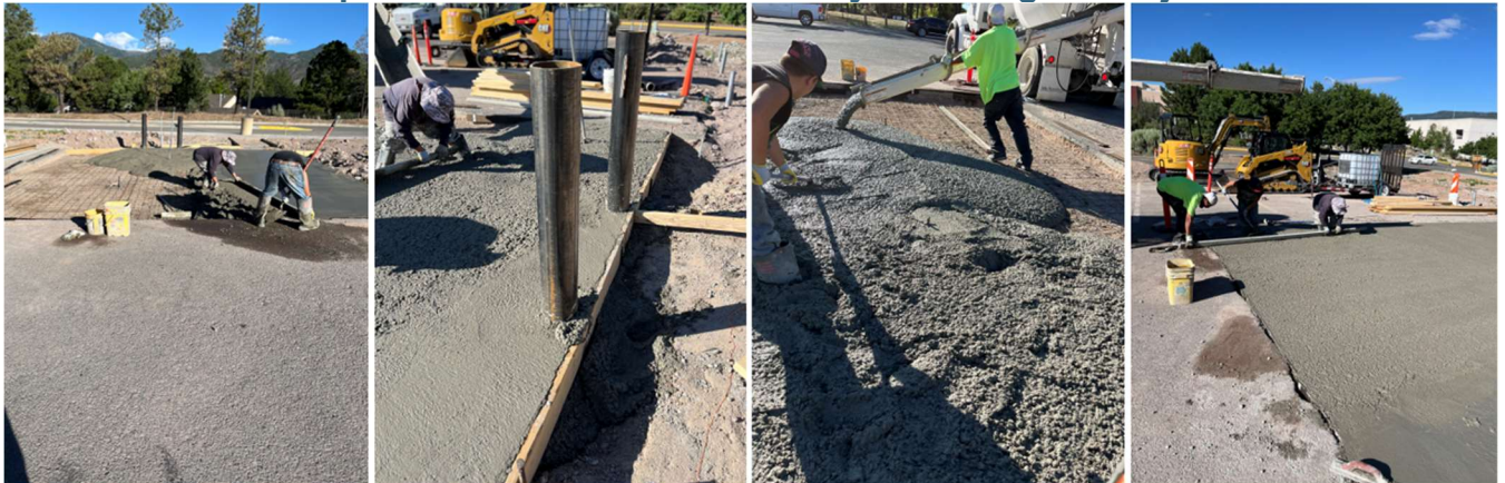
Concrete pour at the Mesa Public Library EV Chargers Project
