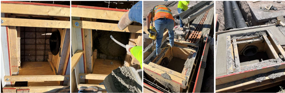
Concrete Pour at the Airport T-hangers Trench Drain Inlet
