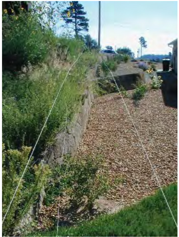
Re-establish trail easement at 35th and Arizona.
