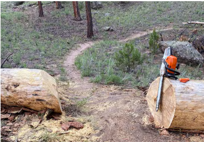
Widen trail tread where necessary.
