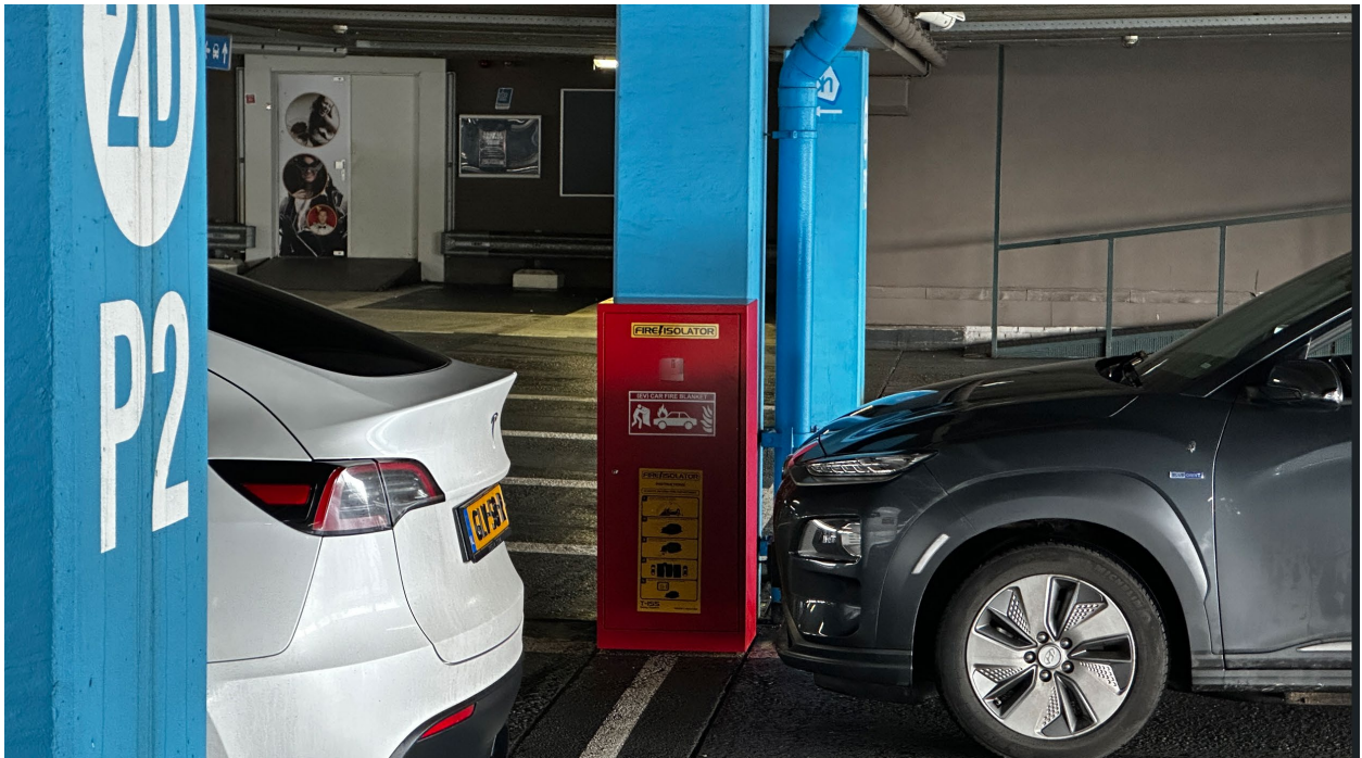
Figure 4-10: Fire isolator cabinet
